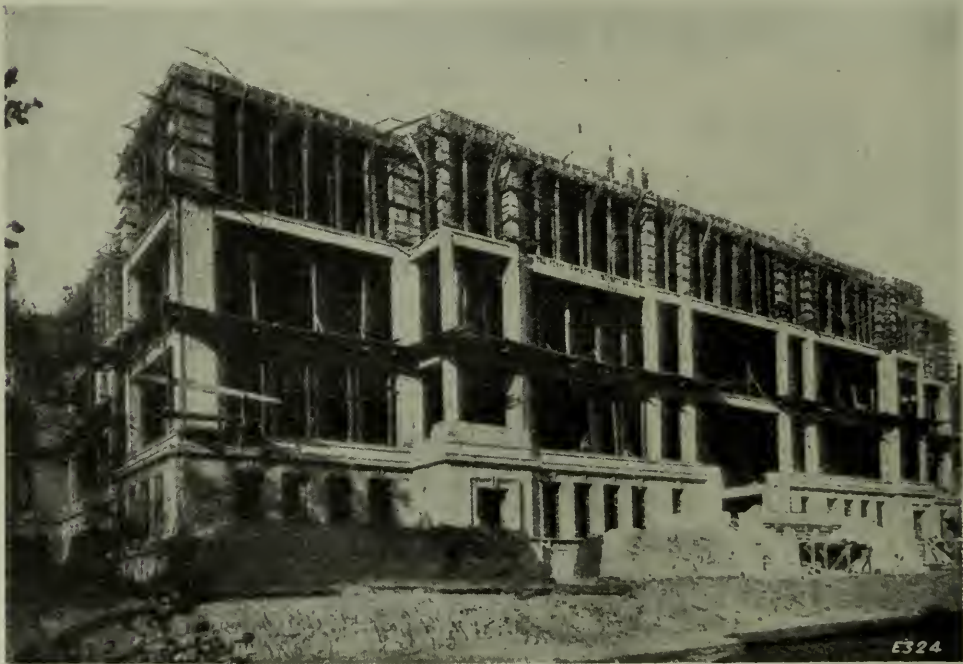
FIG. 7. A SCHOOL BUILDING UNDER CONSTRUCTION.
